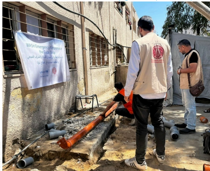
With community members' help, latrine sewage pipes were connected to classroom facilities at the Bachir El Rayes PA shelter in Gaza City, improving sanitation infrastructure in a displacement setting.
