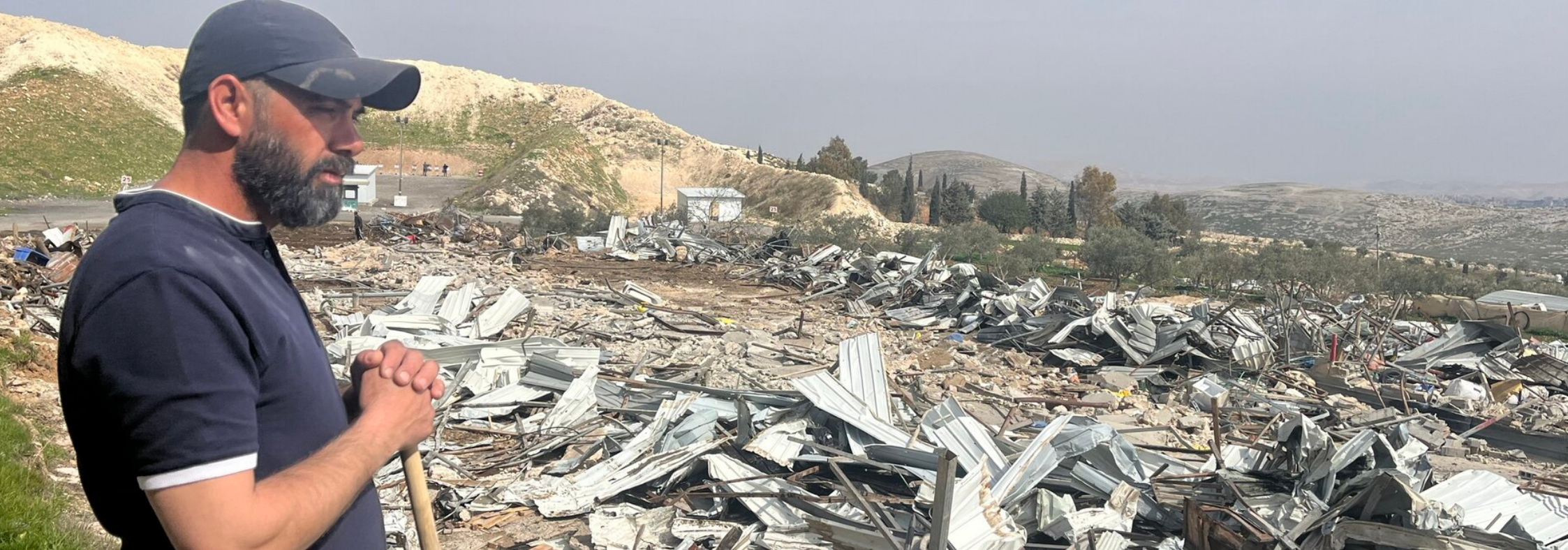
Palestinian observing his destroyed property following the demolition of 12 structures by Israeli forces in Az Za'ayem Bedouin community, Jerusalem, on 3 March 2025. Photo by OCHA
