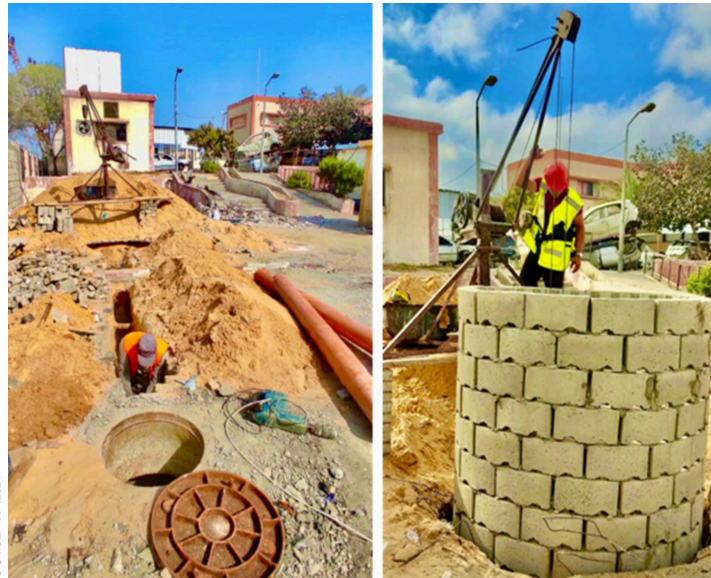
UNICEF supported the construction of four septic tanks at Nasser Hospital in Khan Younis to control sewage overflow.
