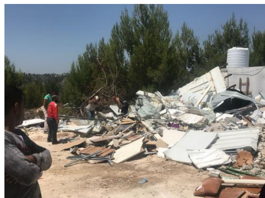
Demolition of residential structure-Al Walja, Bethlehem 25 Aug 202, ©Photo by OCHA
