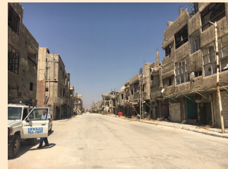
Streets after rubble removal
