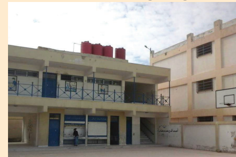
A school after rehabilitation
