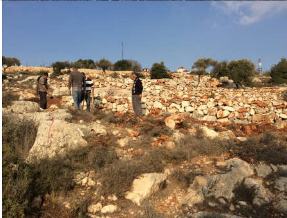
7.3 : Rehabilitation of the Agricultural Dry-stone Walls in the Wadi al- Makrou .
