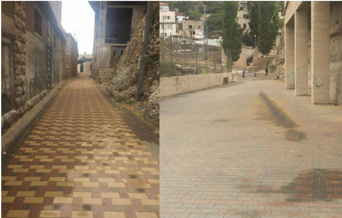
7.2: AL-Medan Square Tiling Works
