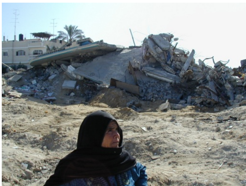
Demolished zone, Rafah camp, Gaza, November 2004.
