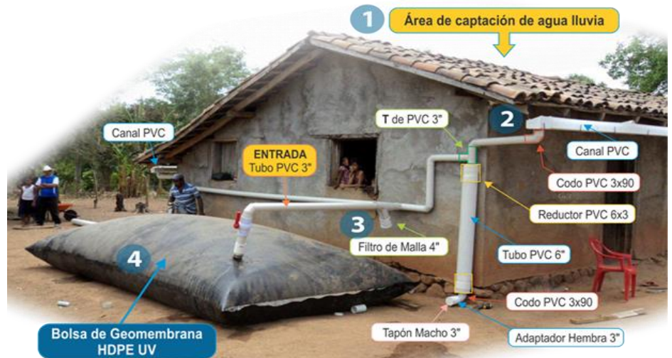
Rainwater harvesting system © PROSADE Lempa CARE Honduras
