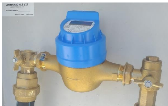
Figure 6: Electronic counter with integrated NB-IoT
