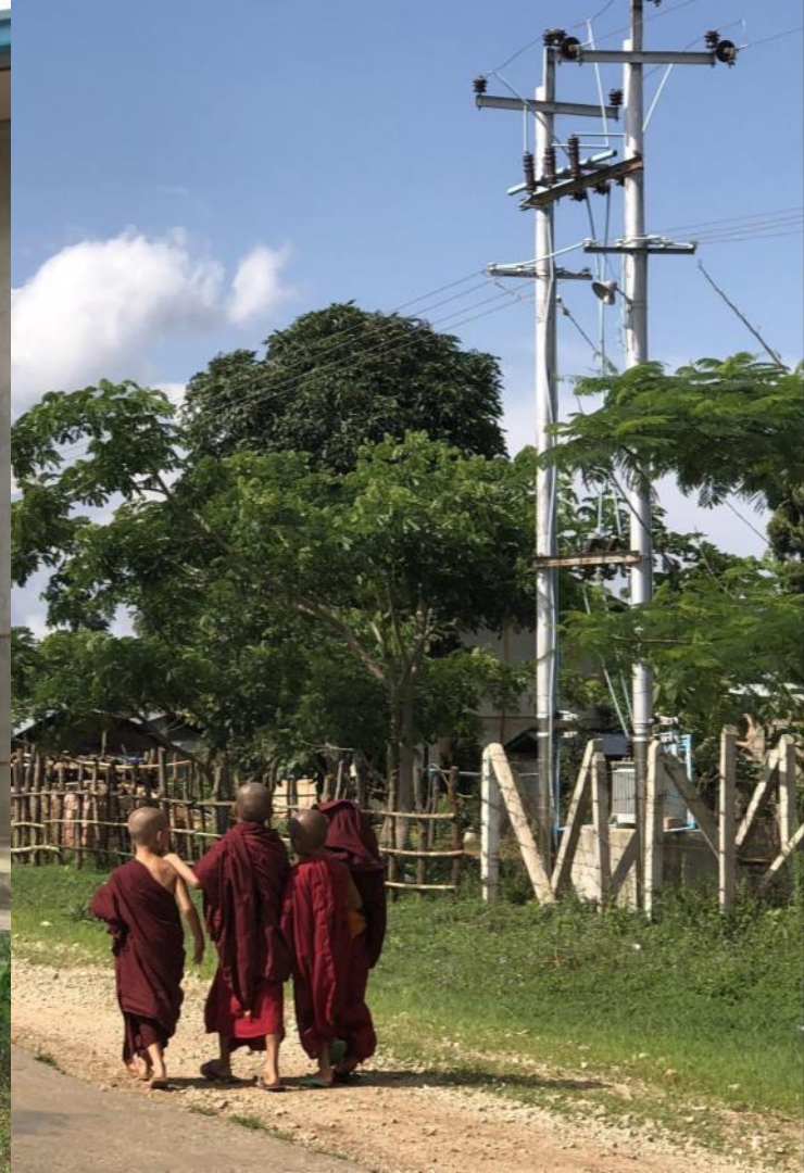
Lin Yuang Chi Micro Hydro Cooperative-Owned Utility in Myanmar Photo Credit: D. Vaghela
