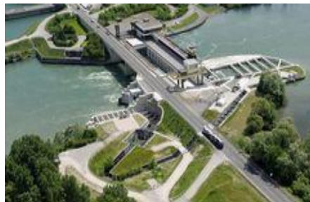
Aerial view of Iffezheim RoR Plant; and Rotor of Turbine 5 (Photos: EnBW/Daniel Meyer-Gerber) from presse@enbw.com
