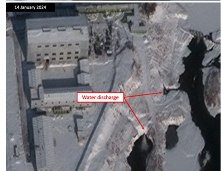
Water discharge from the LWR
