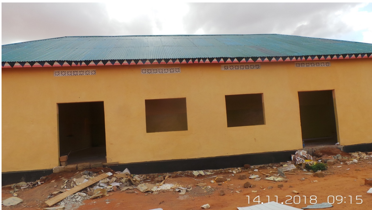
Figure 3 Dollow Airport Rehabilitation
