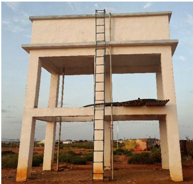
Figure 7: Rehabilitated Cawagle Borehole
