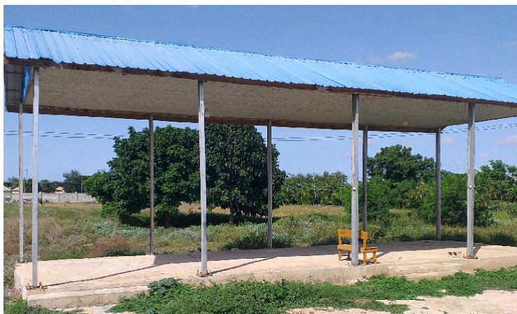
Figure 10: Roofed parking space at Balcad General Hospital
