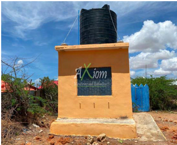
Figure 8: Water kiosk constructed in Beletweyne
