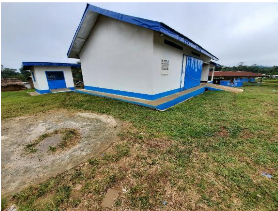
Photo: Newly constructed warehouse in Loguato
