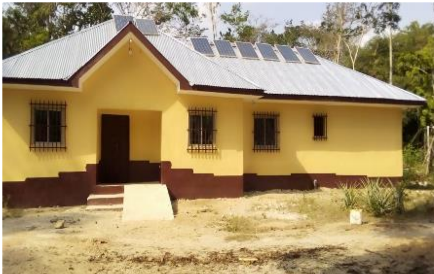
Photo: Newly constructed border post Glio Tempo
