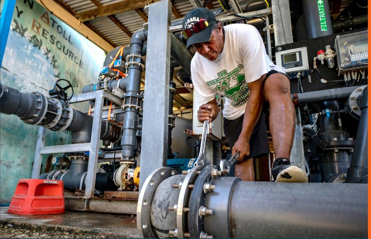
The Ebeye Water Supply and Sanitation Project is linking all households in Ebeye, Marshall Islands to upgraded freshwater and sewage facilities that reduce water leaks and sewage overflows.
