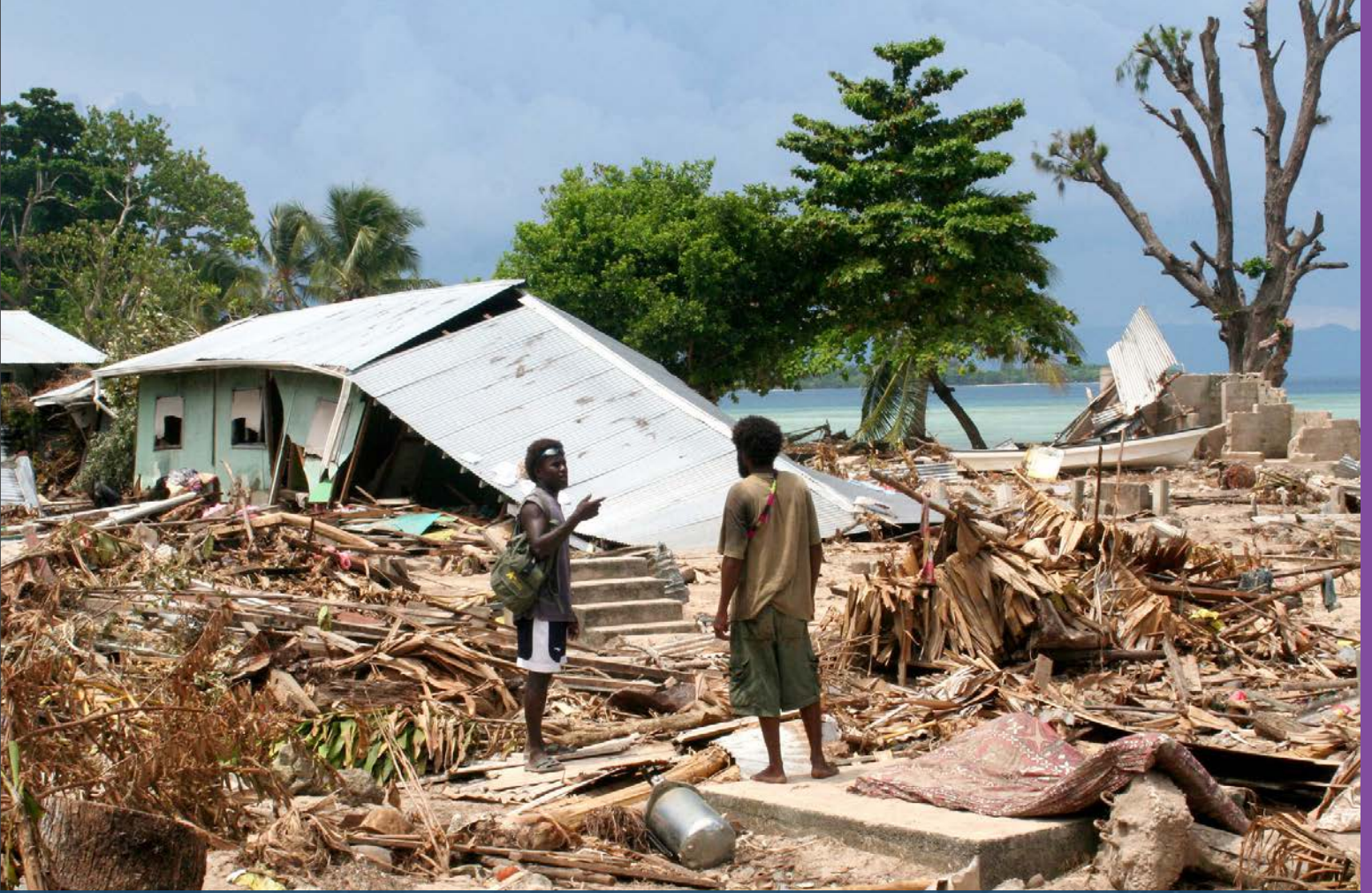
Tsunami damage, Solomon Islands 2007.
