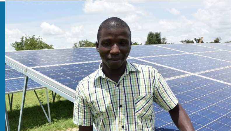
3.6 MW solar mini-grid project in Burkina Faso receiving USD 10 million selected in the third cycle.
