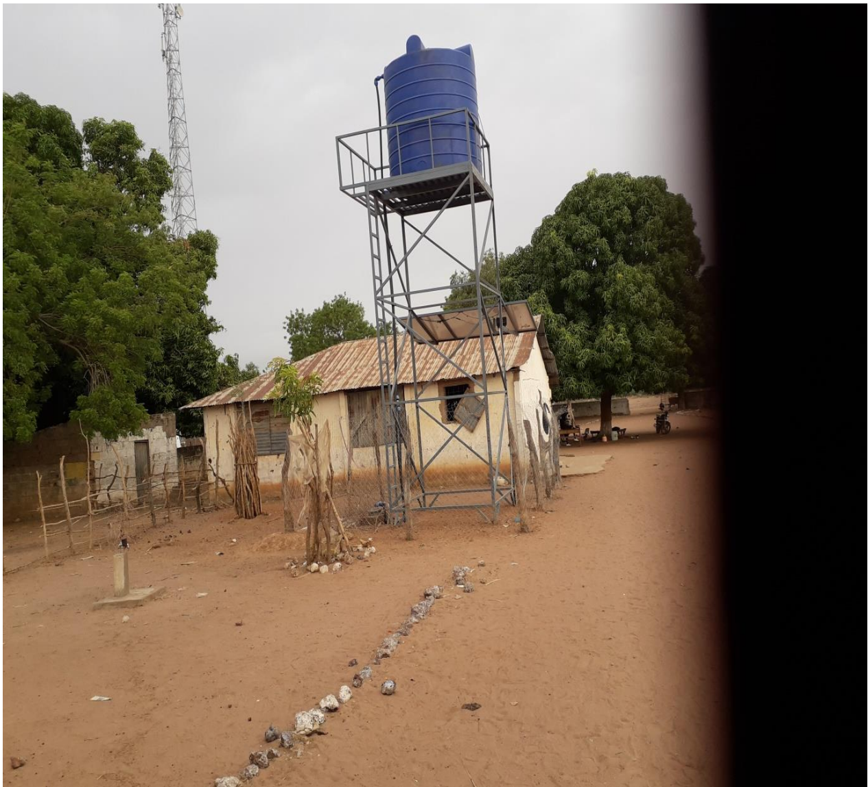
Plate 4: An Improved Village Water Supply System
