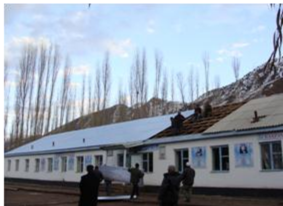
School # 3, Sangvor Jamoat, Tavildara district During rehabilitation works/UNDP Tajikistan
