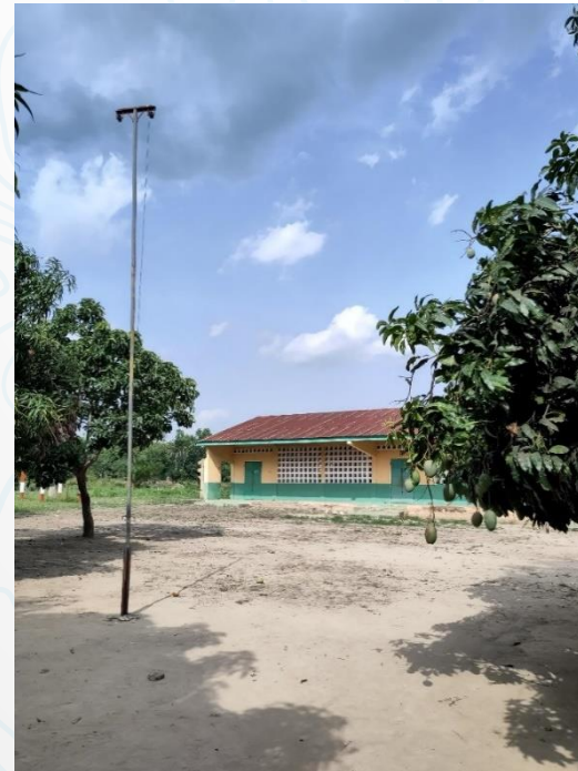
Equipment to survey school location in Togo UNESCO-IIEP, 2023
