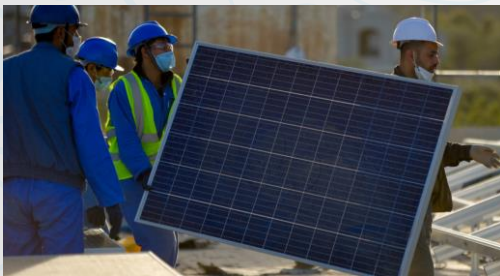
Men install solar panels for a hospital in Yemen UNDP, 2021
