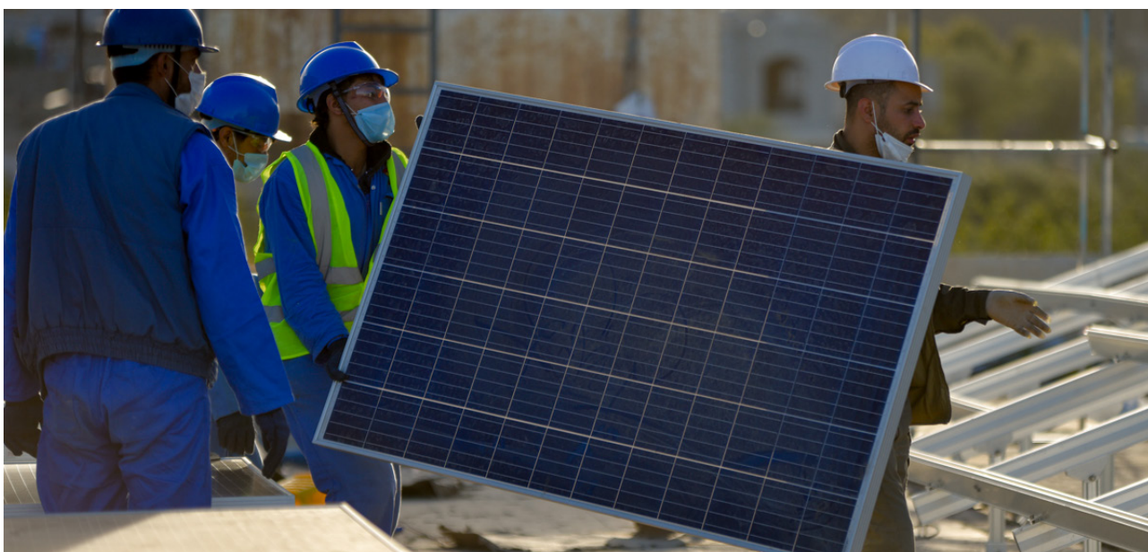
FIGURE 21: Men install solar panels for a hospital in Yemen. UNDP/ 2021
