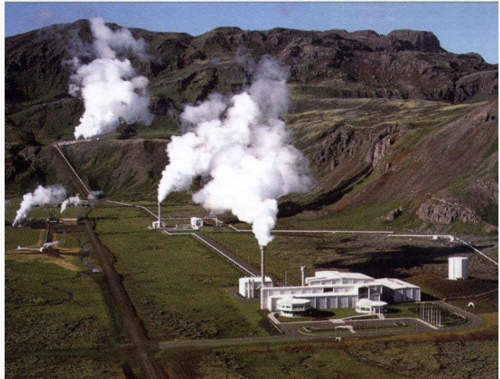
Nesjavellir, Iceland. 300°C fluid used to produce electricity
