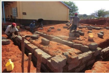
New classroom at Mwatate Secondary School, (Oct 2012)
