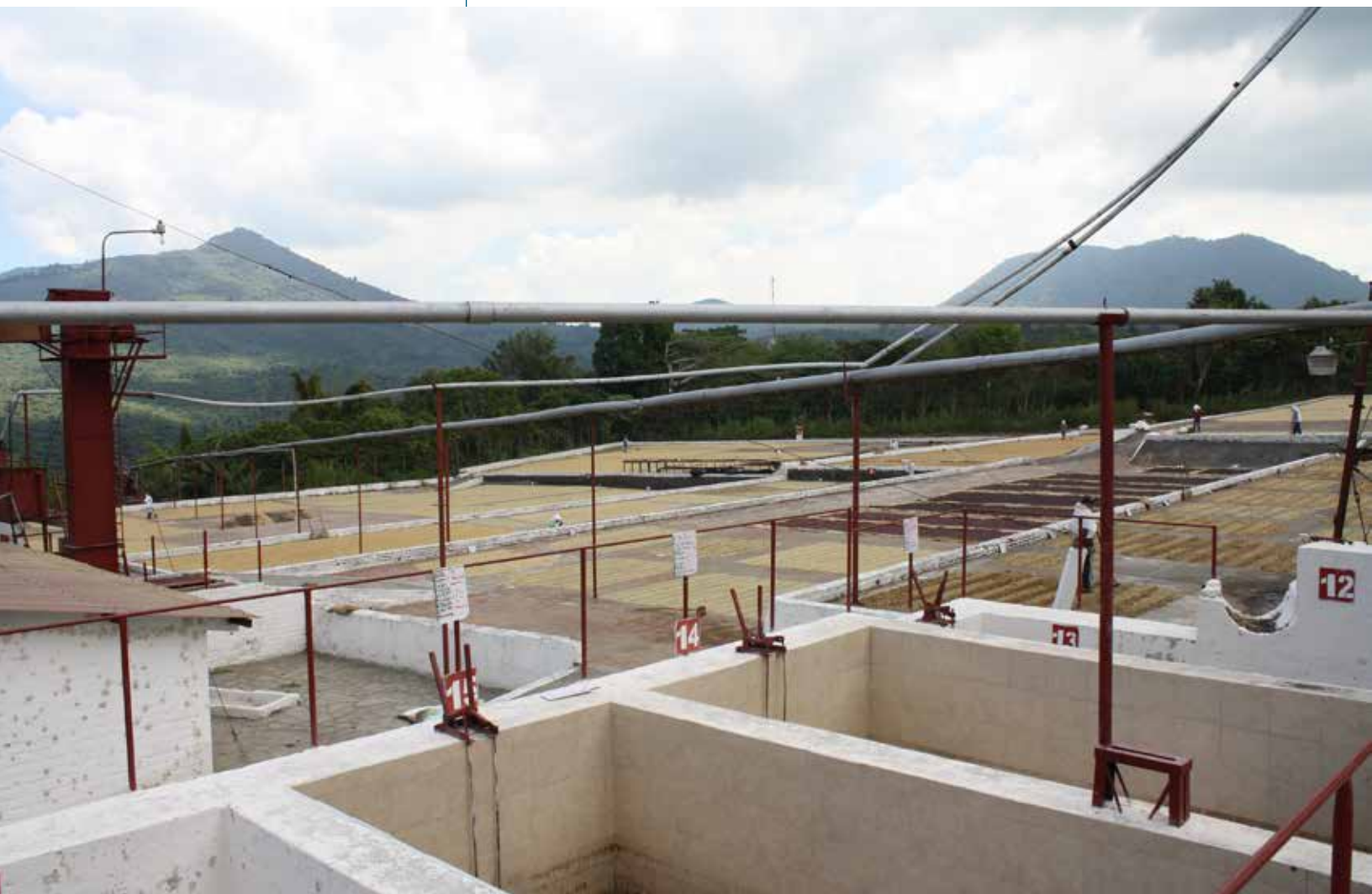
Coffee drying facility in El Salvador. Photo by Seth Shames/EcoAgriculture Partners.
