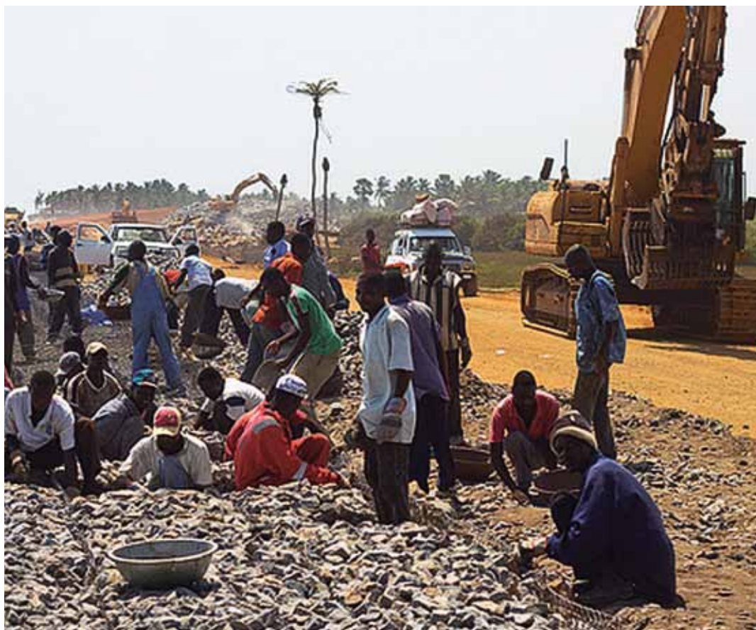
Road construction in Ghana
