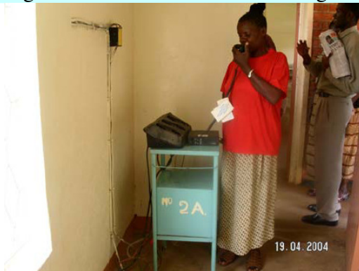
Radio Base Station
