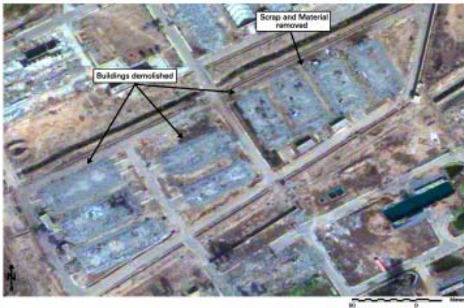
Figure A.5 Dismantled Shumokh store site (22 February 2004)
