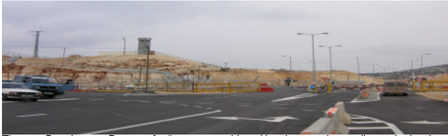
The new Barta'a gate. Passage for 'long-term residents' has improved according to the local mayor.
