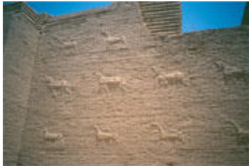
Babylon Temple: update on damage assessment
