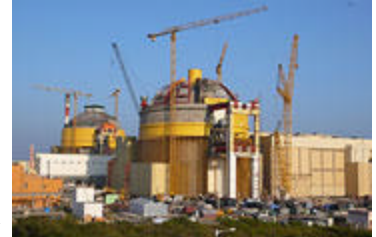
Pressurized Water Reactors (PWRs) under construction at a nuclear power plant
