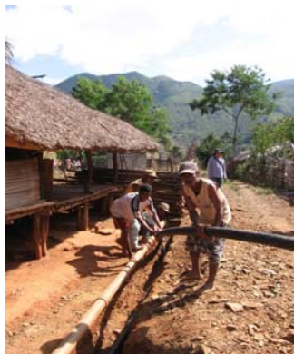
Laying new pipe system in Upper Lacro, Manatutu
