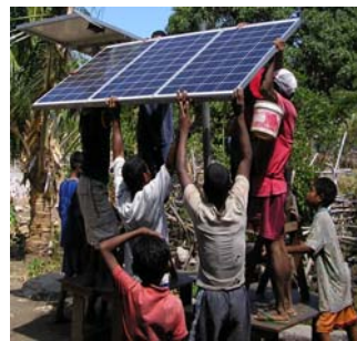
Installation of Community Facility Solar System on Atauro Island.
