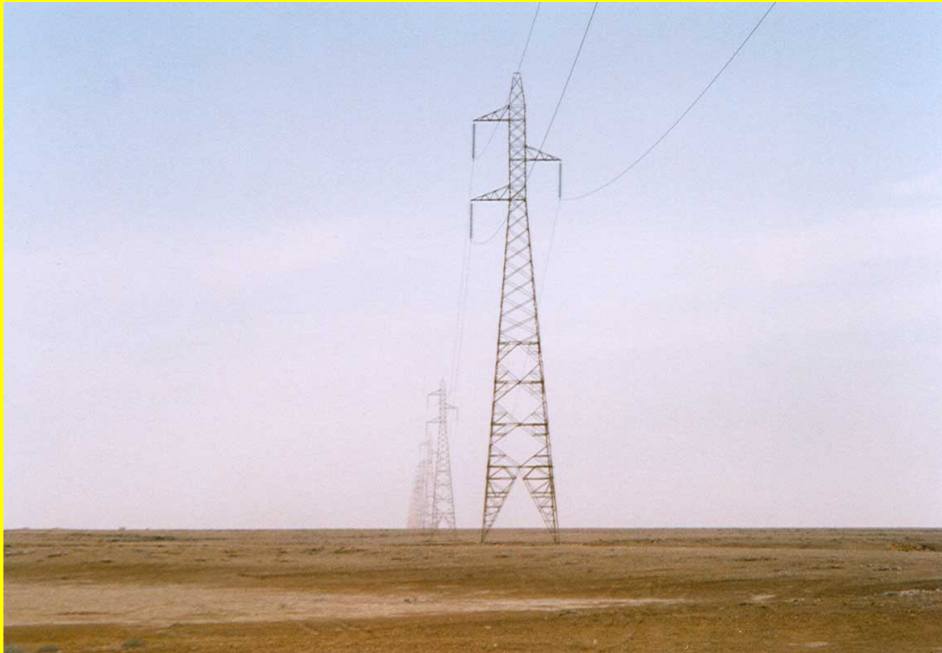
225 kV public ONE grid line heading North, 20 km away from Tarfaya
