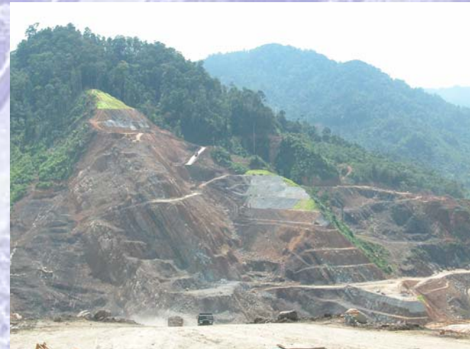
Hydro-seeding and slope protection immediately after excavation
