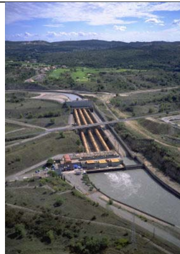
Figure 7: Mallemort power plant along Durance river
