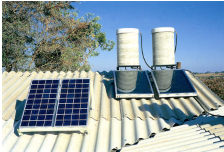
fig. 3: Solar water heating systems and the photovoltaic unit at the Chitungwazi Clinic
