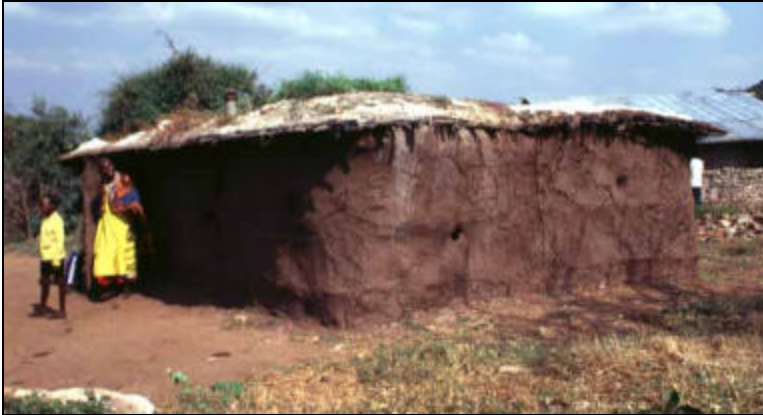
Figure 1 (above): a traditional Maasai house, showing squat construction and tiny windows. The flue was fitted some years previously in a local government initiative, but no longer works (see
