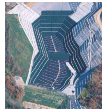
The biggest landfill facility in Japan
