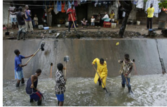
UNMIL Special Engineering Projects provide employment for skilled and unskilled labourers
