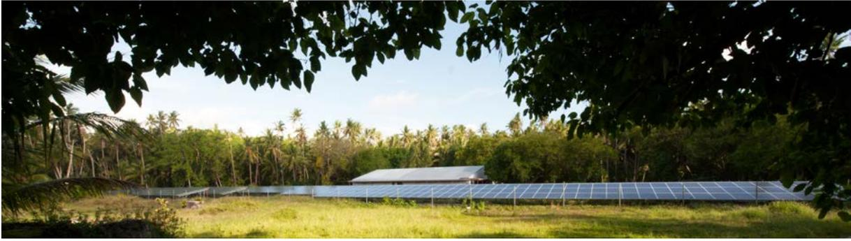
This large solar photovoltaic/diesel hybrid mini-grid system, installed on Fakaofa, one of the three atolls that make up Tokelau, delivers over 90% of the atoll's electricity needs from renewable sources.
