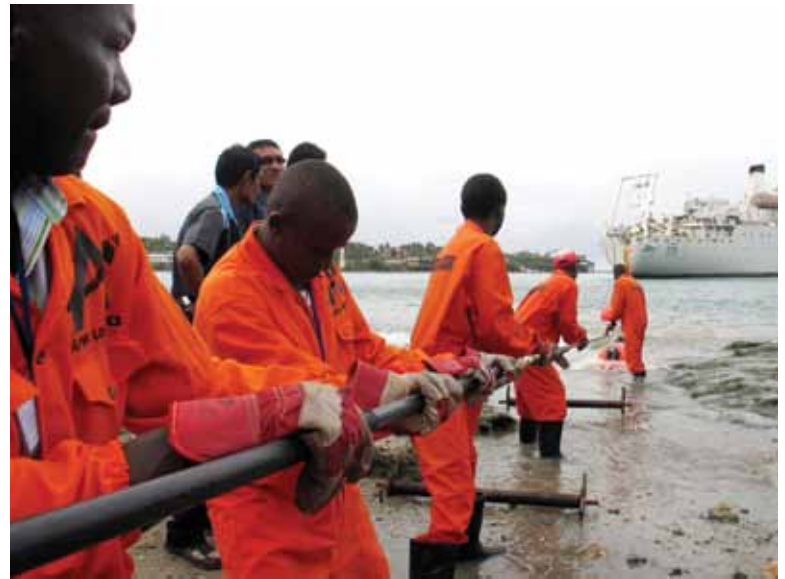
Laying fibre-optic cable off the East African coast: More least developed countries will have faster and cheaper communications links with the outside world. Photo: Reuters/Joseph Okanga
