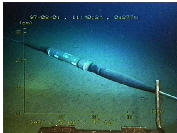
Cable In-line OBS on the 1277m depth of seafloor
