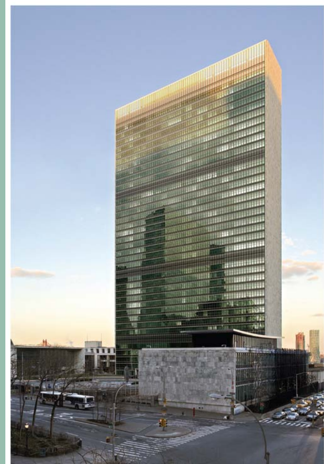
New Double-Glazed Curtain Wall
