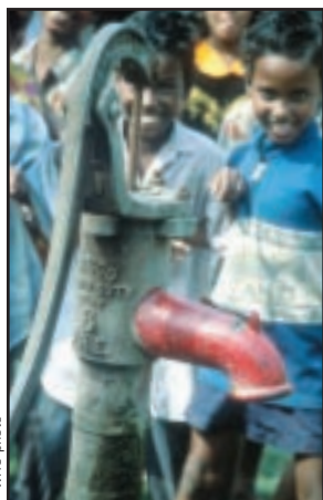
A red painted pump means "don't drink this water".
