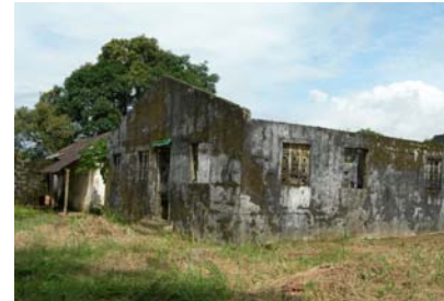
Soul Clinic Police Depot before renovation
