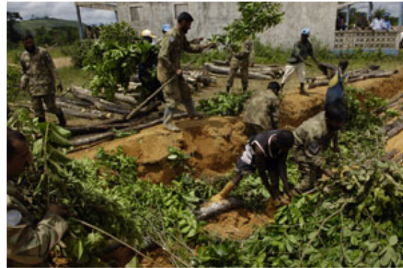
Pakistani contingent demonstrates how emergency road repairs are carried out
