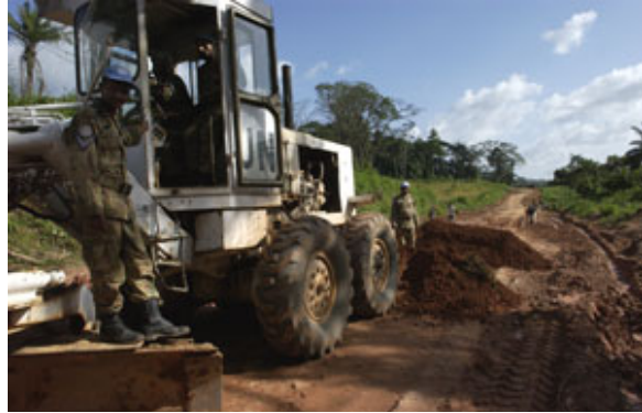
UNMIL Pakistani engineers at work on the Voinjama-Zorzor road
