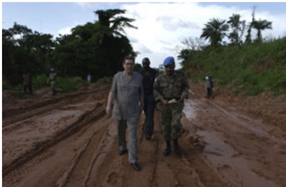
SRSR Doss inspects the road work near Voinjama
