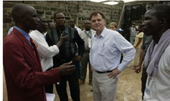
DSRSG Ryan with Rivercess Superintendent and Senior Senator inspect the renovation work at the City Hall
