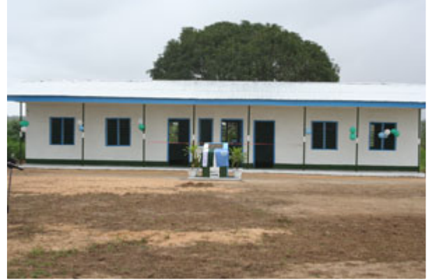
New school building commissioned by the UNMIL Nigerian contingent
