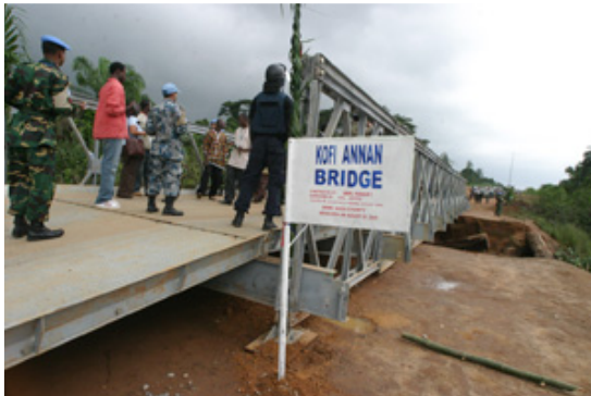
The Kofi Annan Bridge constructed by UNMIL’s Pakistani Engineers
